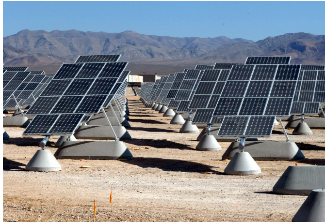
Figure A.1: Crystalline silicon solar cells in the Nellis Solar Cell Planet, located within Nellis Air Force Base in Nevada- US. Photo source is [10]
