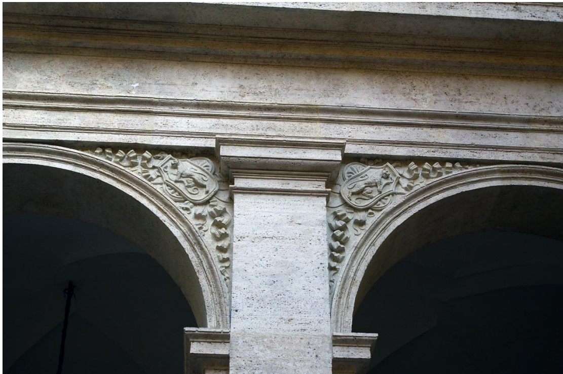
Abb. 48: Palazzo Ruggieri, Innenhof, Loggia, Erdgeschoss, Detail
