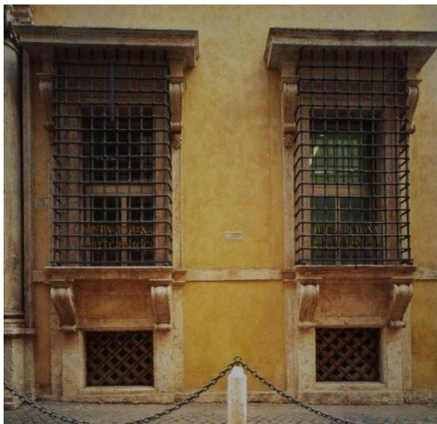
Abb. 21: Palazzo (Maffei-)Marescotti, Fassade, Erdgeschoss, Detail
